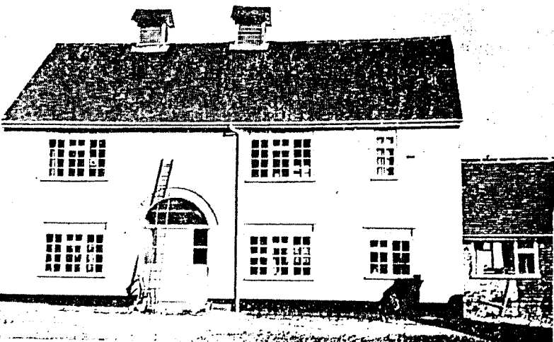
Right: the old brewery at Rowsham, Buckinghamshire, now converted to a private house (photograph above).
